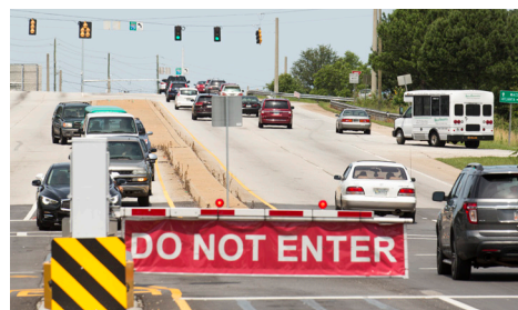
A series of warning gates are placed along every entry to alert motorists prior to the point of entry that the access is closed.
